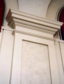
Detail of a column cladding made of Acrystal Prima and laminated with quadriaxial 200-4D fabric of 7 mm thickness
